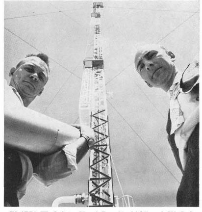
IN AREA III, designer Marcel Reynolds (right) and Sid Cook stand in front of 300-ft. drop tower which supports Zero G facility tube inside the structure. Instrumentation package which Sid holds is dropped down the tube during tests. "Tee" connection from tube leads to 1000 cu. ft. vacuum tank and turbo blower.
